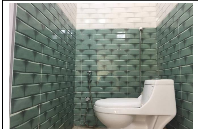
2-Accessible toilet, College of Administration and Economic
