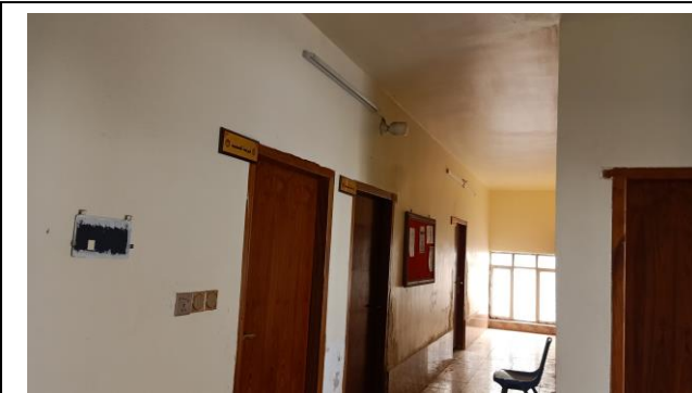
3- Shutting down of the electrical devices after the work hours
