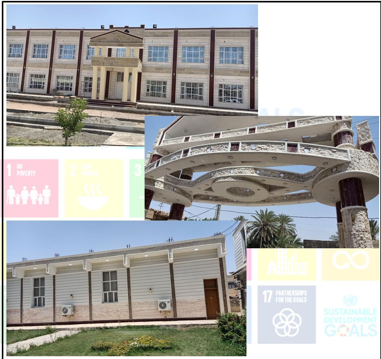
Plate 2: Example of new buildings in UOS faculties.
